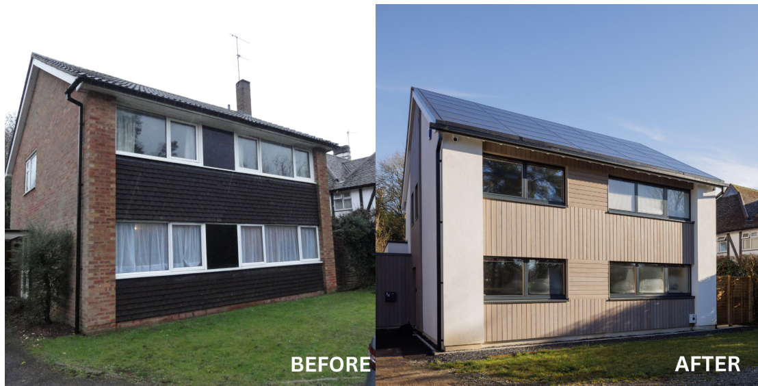
Fig. 1: Harpenden EnerPHit Plus, UK Passivhaus Awards finalist 2023
