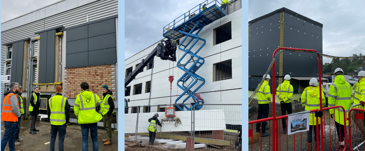
Fig. 16: From left to right: 1) Steel rig at BE-ST campus. 2) Panel install at Faifley Campus. 3) Test rig for Faifley Campus. Image credits: Morrison Construction.
